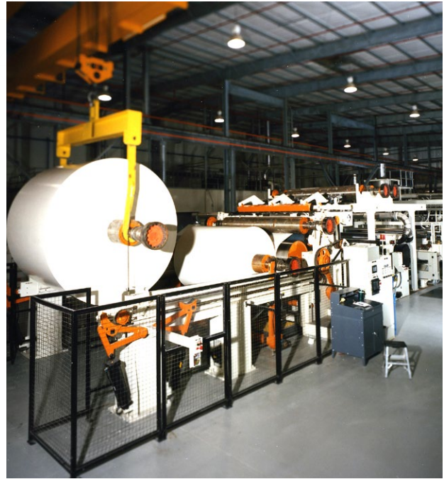
Board Coating Line
